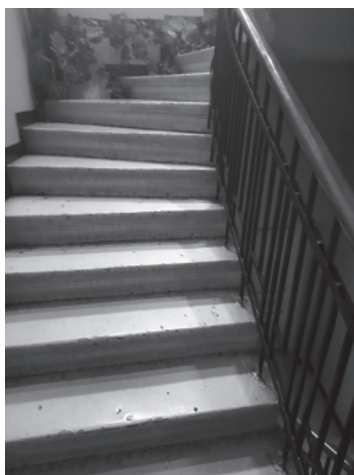
The stairway in Aleko's house.
